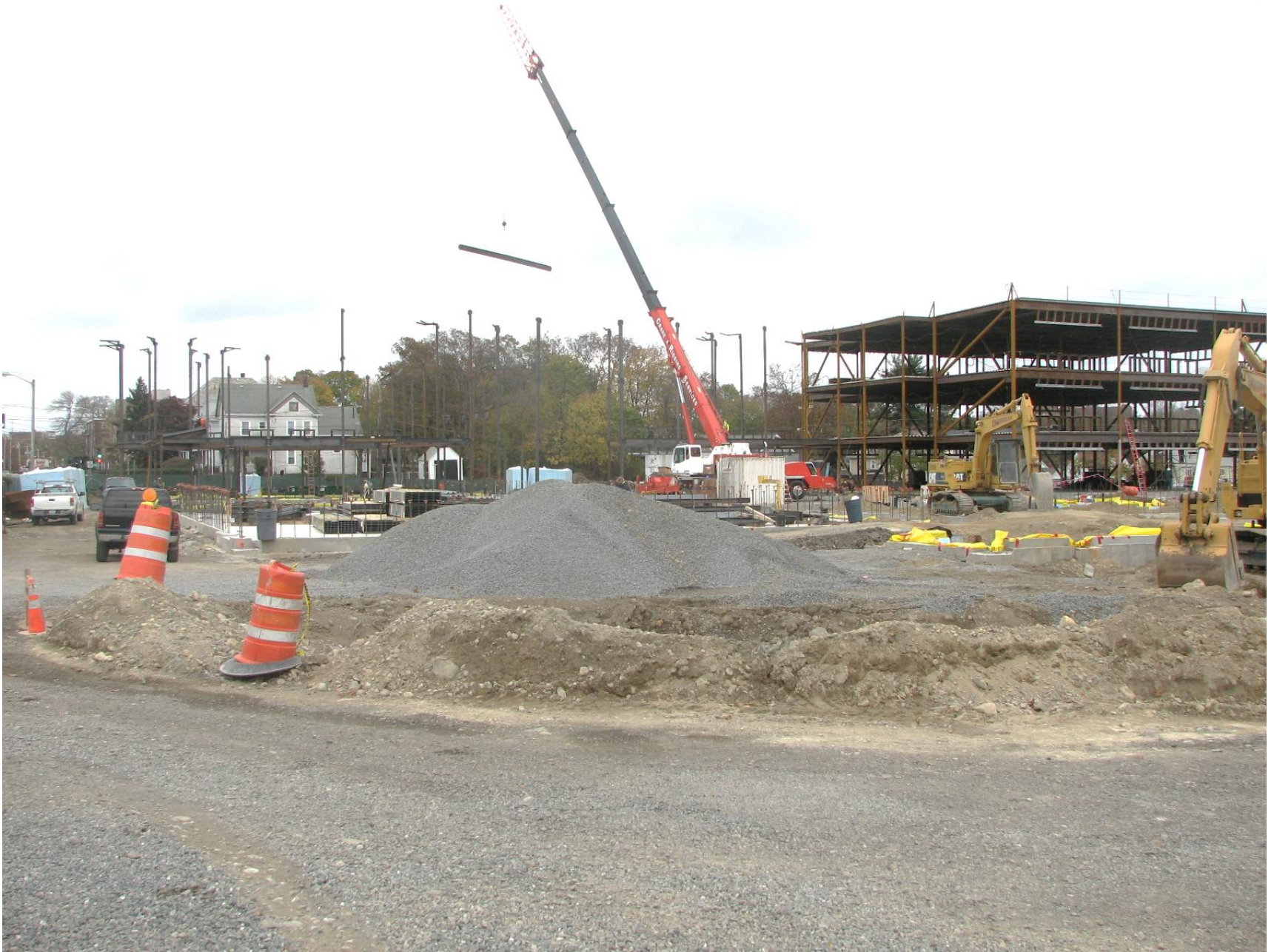
Building Site Overview
