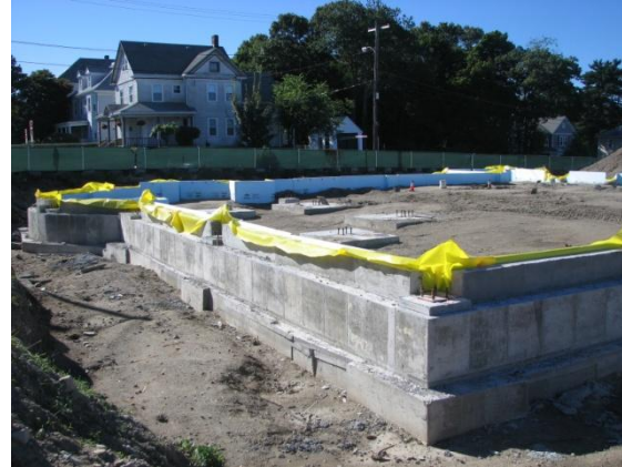
Administrative Offices Foundation
