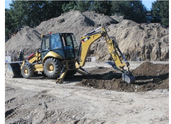
Excavation for Auditorium Foundation
